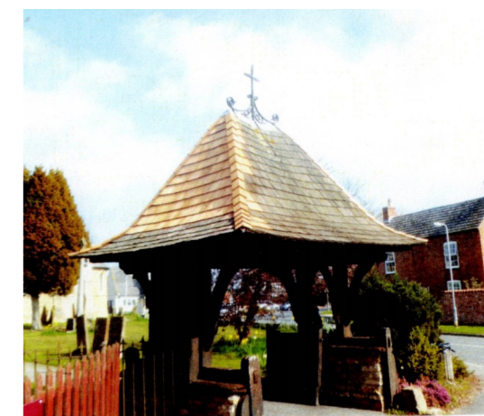
Swinderby All Saints. Assorted relatively minor fabric repairs to the wooden shingle roof on the lychgate and stonework repairs to the Porch. The work was completed in April 2012.
