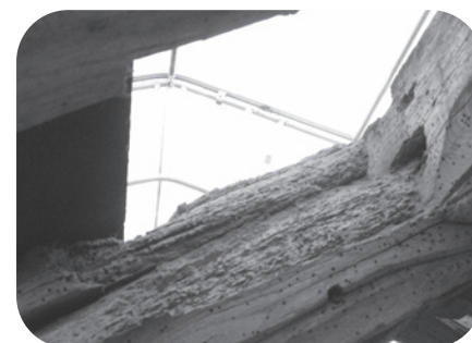
Roof repairs in progress at Grimoldby, (near Louth) St Edith. Grimoldby.
